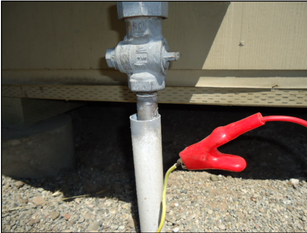
Figure 2. Conductive (Tracer Wire)
