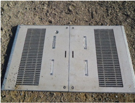
Primary Enclosure (QEW required for entry)
