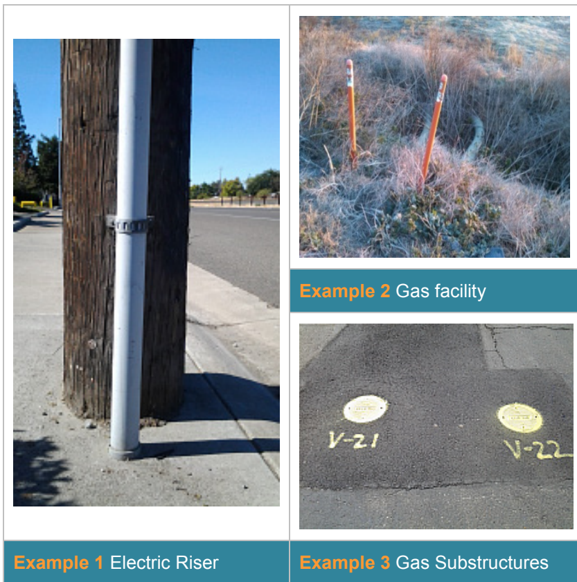
Figure 2. Examples of Visible Facilities That May Conduct Signal
