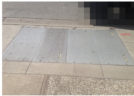
Primary Enclosure (QEW required for entry)
